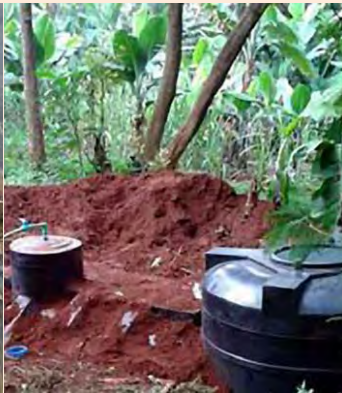
Photo: Blueflame Water and Energy Solutions
