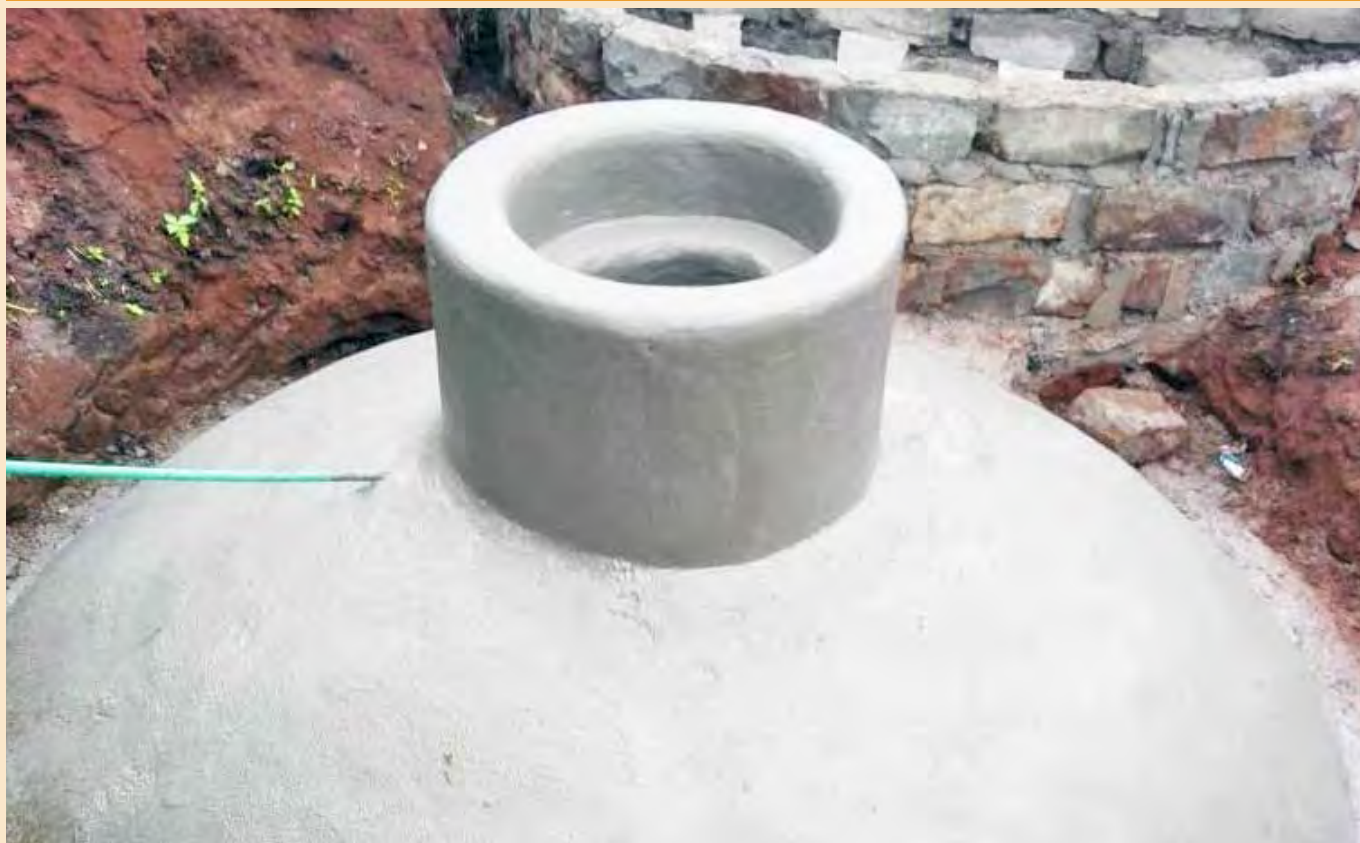
Photo: Blueflame Water and Energy Solutions
