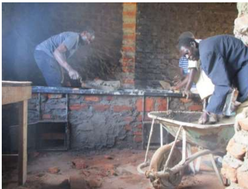
ICS construction in Nebbi district
