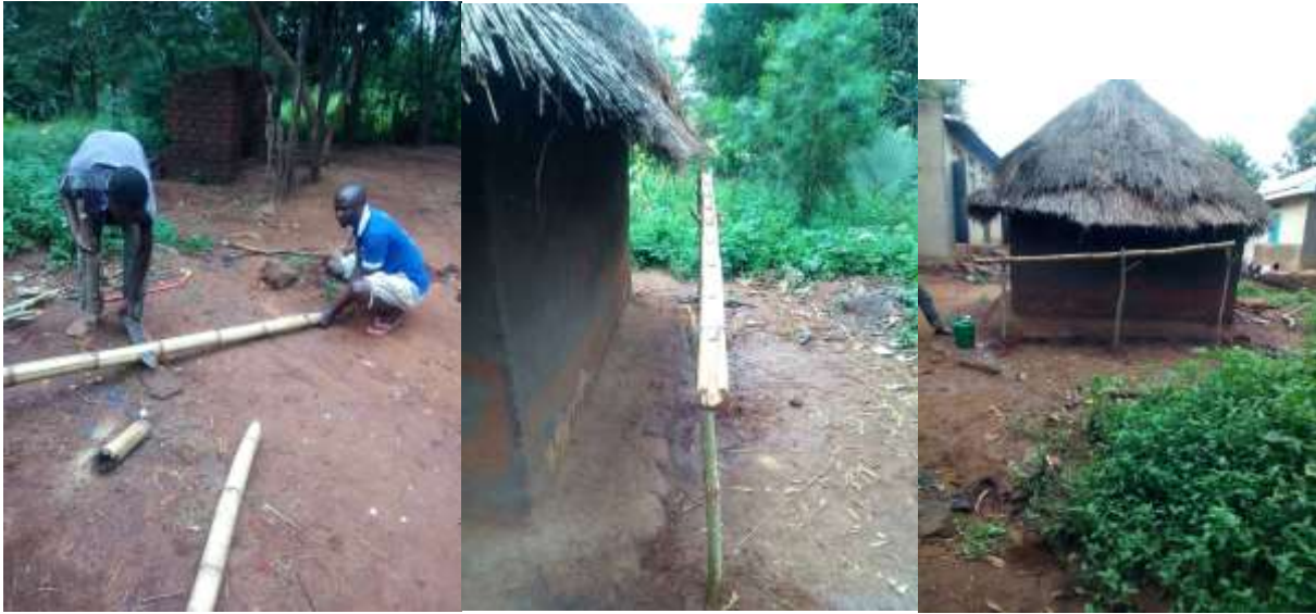
L-R: Field staff Nebbi during the demonstration of water harvesting from grass-thatched houses using bamboo as a water gutter.
