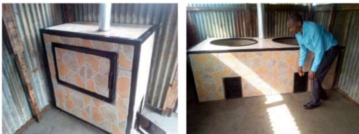
Figure 32: Newly constructed baking oven (left) and institutional cookstoves (right) in South Sudan. Photos by JEEP.
